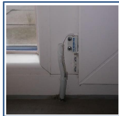
Figure 3-15: Window open/close sensing contact with wiring
