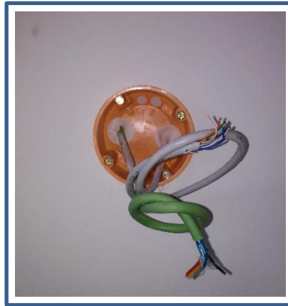
Figure 3-14: Wall box with European Installation Bus (EIB) and FTP cabling to host a wall switches, digital inputs from a door contacts and a room thermostat
