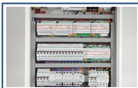
Figure 3-11: BACS hardware mounted on a DIN rail in an electrical control cabinet
