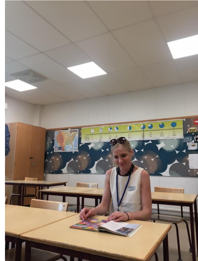
After: New LED fixtures
