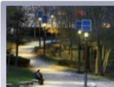
Solar photovoltaic systems
