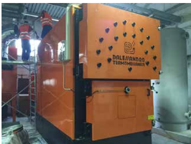
Project visit Burgas, September 2016 – new heating system in the central for several school buildings (from diesel fuel to pellets) – project soon to be finished
