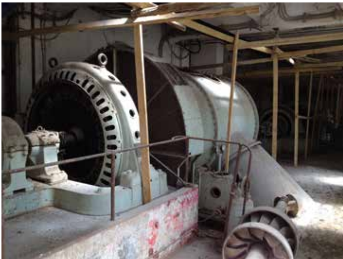
Intake reservoir, small spillway in the intake canal and turbine hall at the old powerstation from the late 1930s
